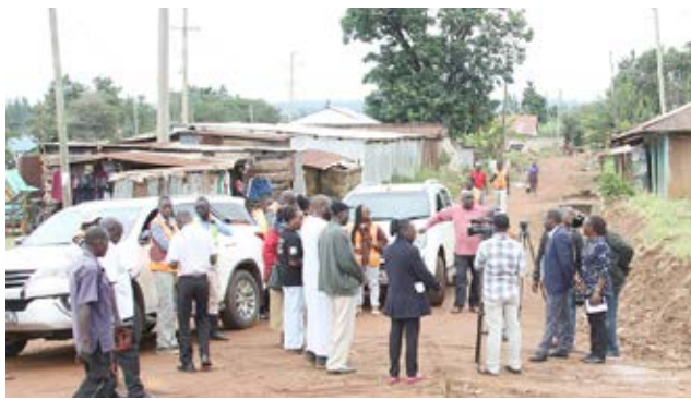
The KISIP team engages with Lukoye SEC members at the Isbatva-Lukoye loop that is set to be tarmacked under the Kenya Settlement Improvement Project (KISIP). PHOTO: GEORGE KAIGA, KNA.
